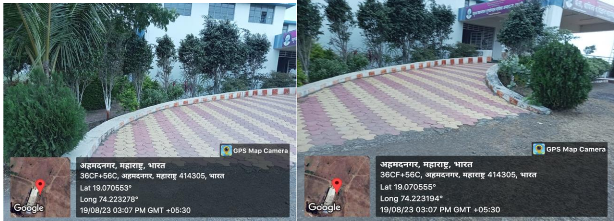
Ramp for disabled students
