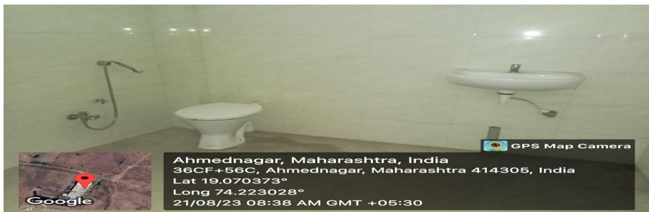
Washroom for Physically disabled students
