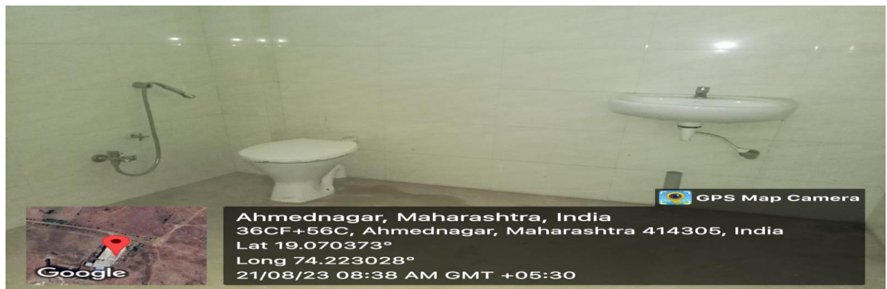
Washroom for Physically disabled students
